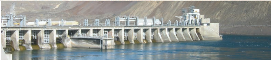
Rock Island Dam Hydroelectric Facility located on the Columbia River, Washington, USA
