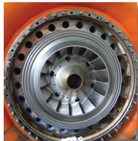
ThorPlas bearings installed in Francis Turbine at Tuai Power Station, New Zealand
